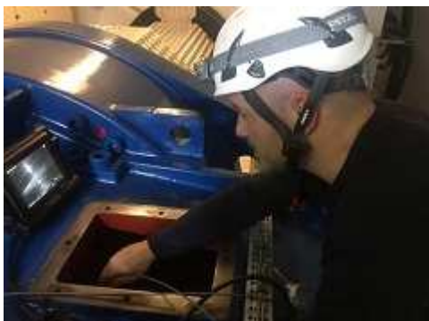
Figure 3: ALL NRG inspector Danijel Bogojevic carrying out a gearbox inspection with the IPLEX RX.
